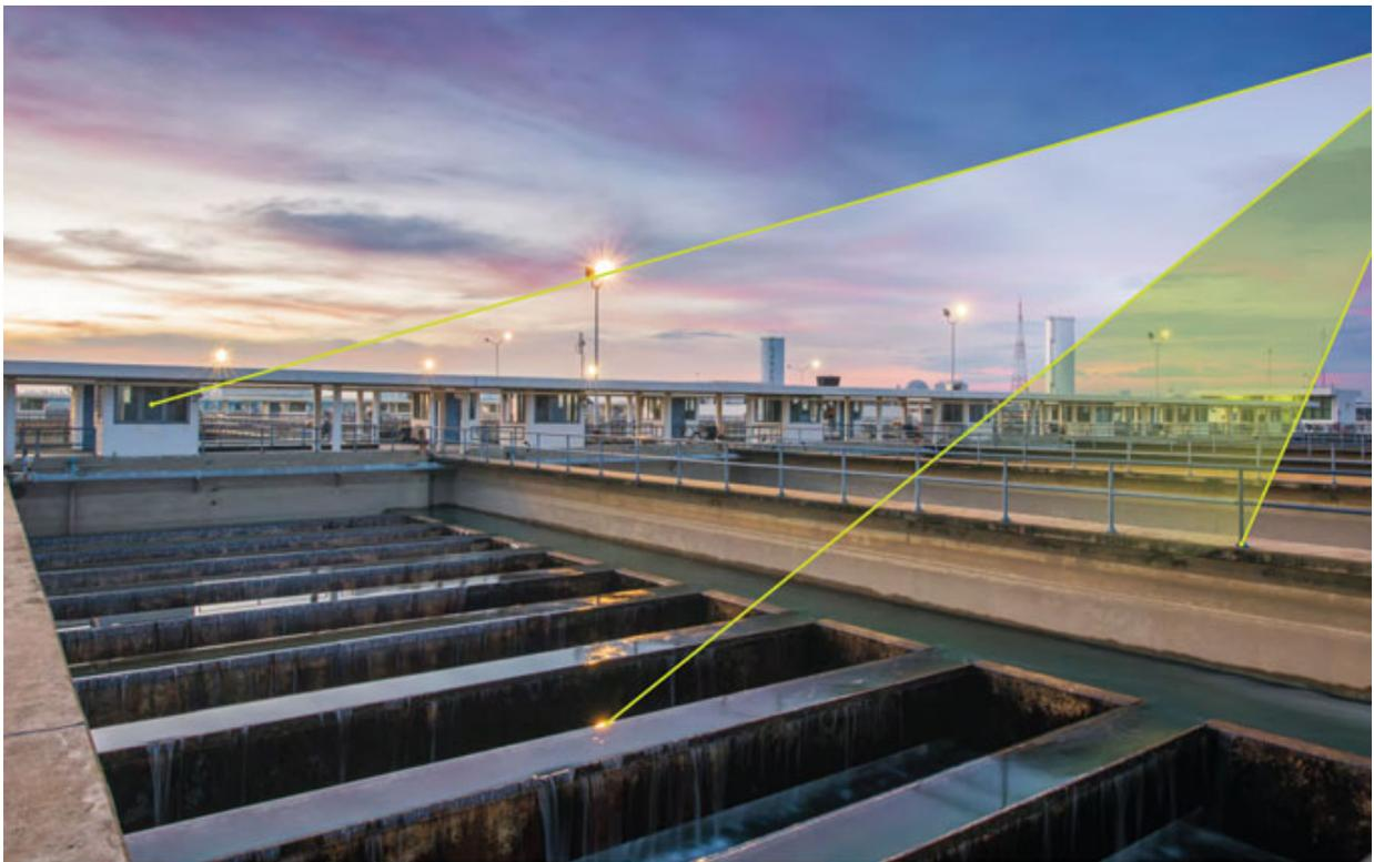
Sand filtration tank at water treatment plant
